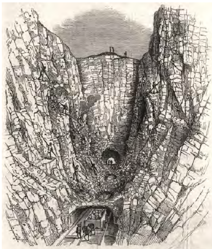
Figure 40. ‘The Rose Hill cutting’ from The Illustrated London News (June 6, 1846 page 388). A tunnel was bored along the line of the route then four vertical shafts sunk from above.
