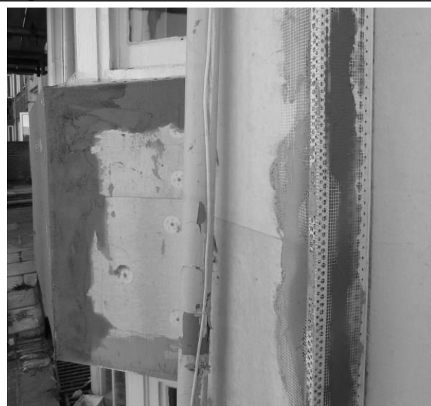
3 Brewer Street's external cladding during installation.
