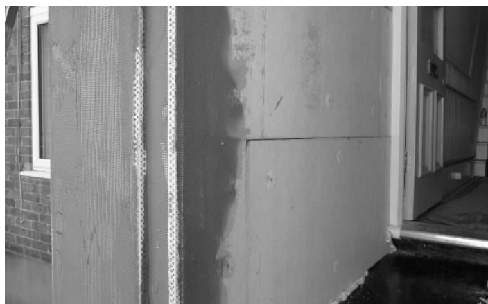
3 Brewer Street's external cladding during installation.
